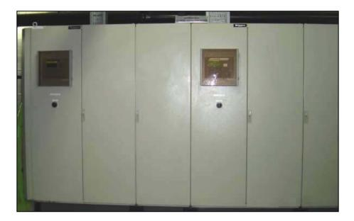
The Thor system has been specially developed to control and monitor cathodic protection systems in plant areas where multiple systems are installed.
